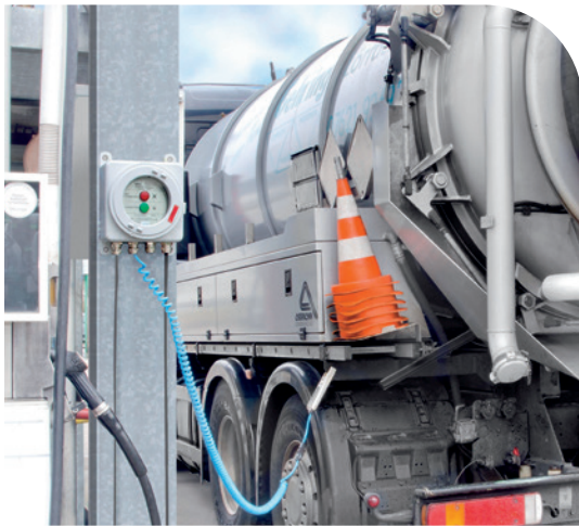
Active Erdung an Tankwagen
