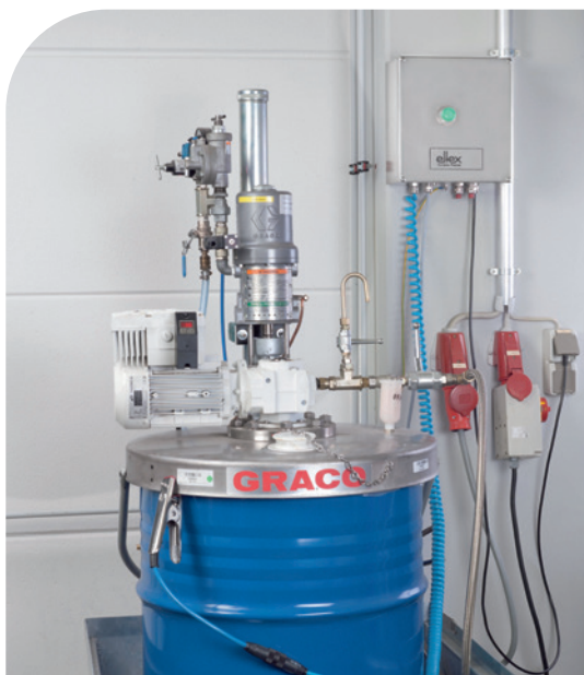
Process safety with Eltex grounding devices in the pharmaceutical industry
