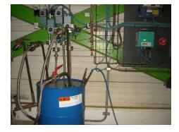
Photo: Barrel grounding with **TERRA**BOX
